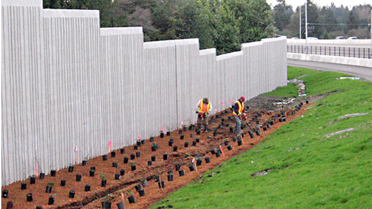
Figure 1 - Construction of vegetative swale in Washington State (top photo and above). Photos courtesy of Craig Cogger, Washington State University
