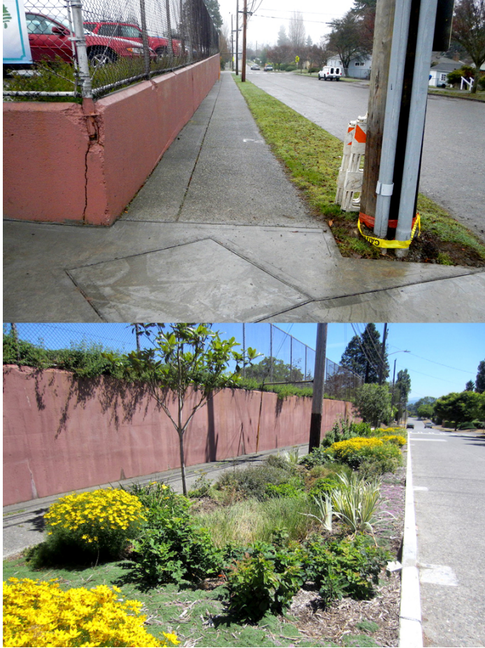
Figure 3 - Biofiltration strip constructed in King County, Washington — before (top) and after (above).
