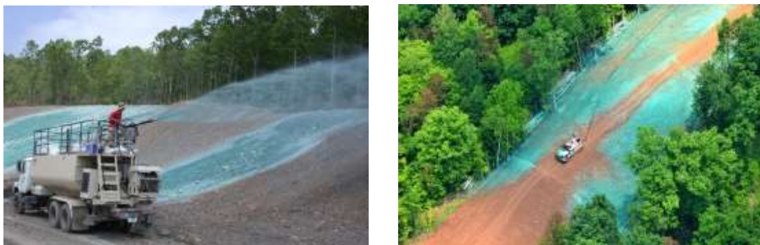
Figures 4 and 5. Hydroseeding following reclamation on a natural gas well site 1 (l) and natural gas pipeline right-of-way 2 (r). Photo reprinted with permission from Jeff Skousen 1 , West Virginia University Extension Service, and Amir Hass 2 , West Virginia State University.
