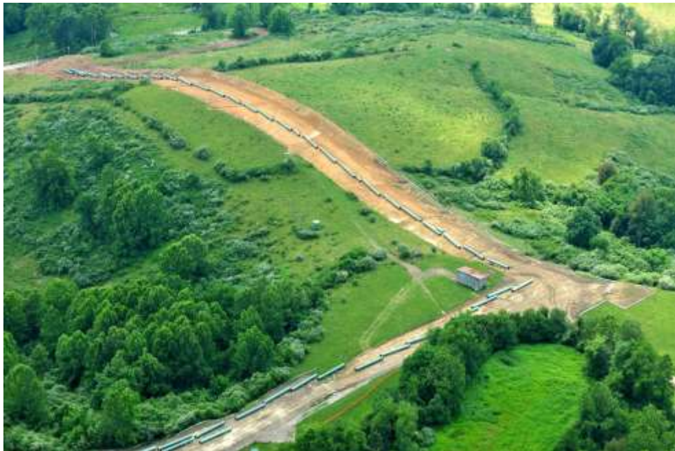
Figure 2. Cleared corridor for natural gas pipeline. Photo reprinted with permission from Amir Hass, West Virginia State University.
