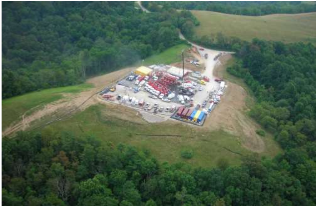
Figure 1. Typical Marcellus Shale well site in West Virginia. Photo reprinted with permission of West Virginia Department of Environmental Protection.
