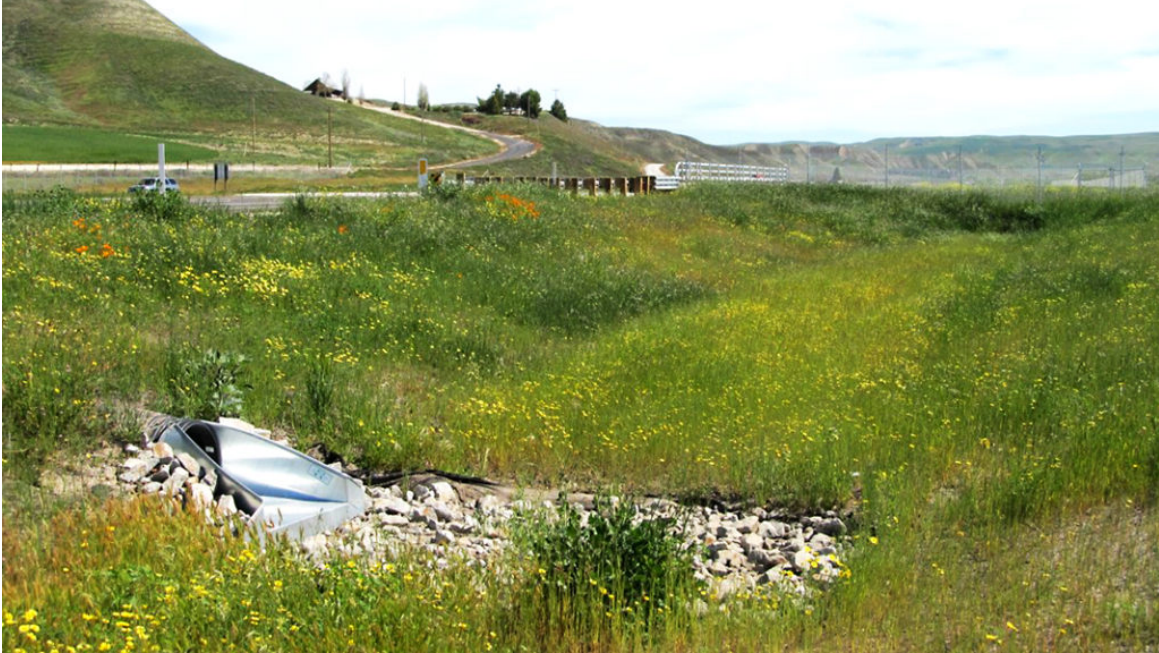
Figure 2 - Bioswale on right of way
