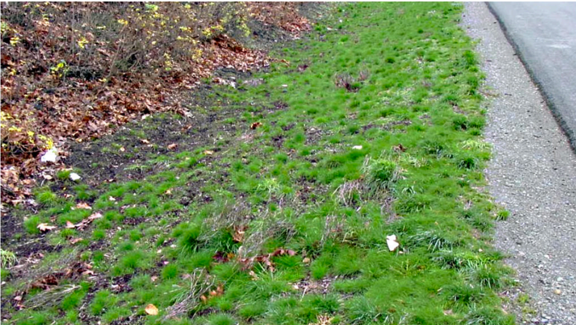
Figure 3 - Compost amended vegetative filter strip. Photo courtesy of WA State DOT
